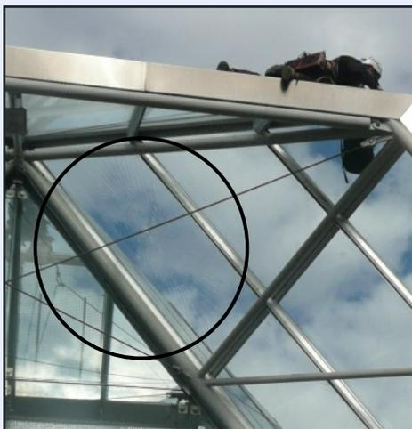
Frost is thought to have caused shattering of a glass panel at the front of the Conservatory
